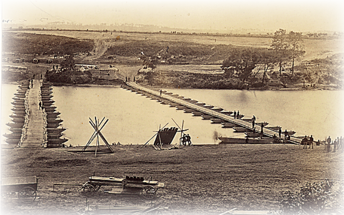
Pontoon bridges across the Rappahannock River at Fredericksburg, 1863
